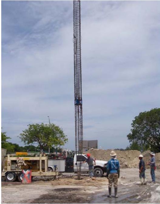
Figure 5 – Installing rebar cage
