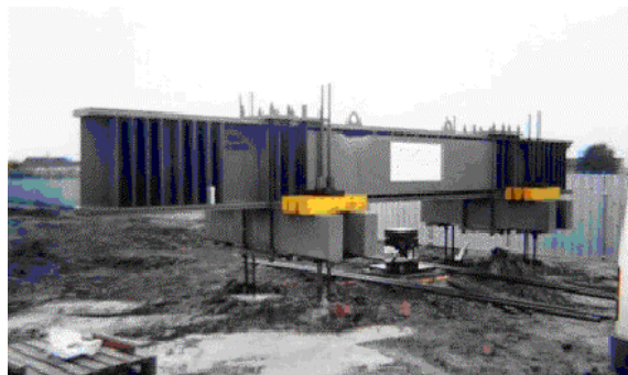
Figure 5. 5.5MN CRAFT set up on 4 anchors with 8 Dywidag bars
