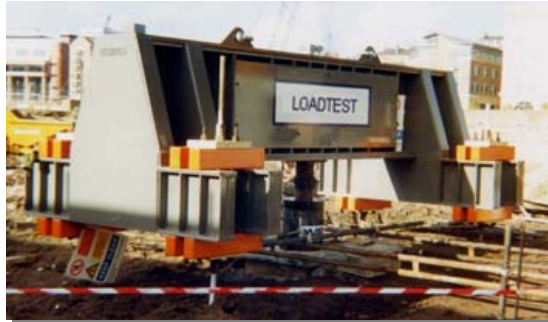
Figure 4. 4 MN CRAFT set up on 4 anchors with 4 Dywidag bars
