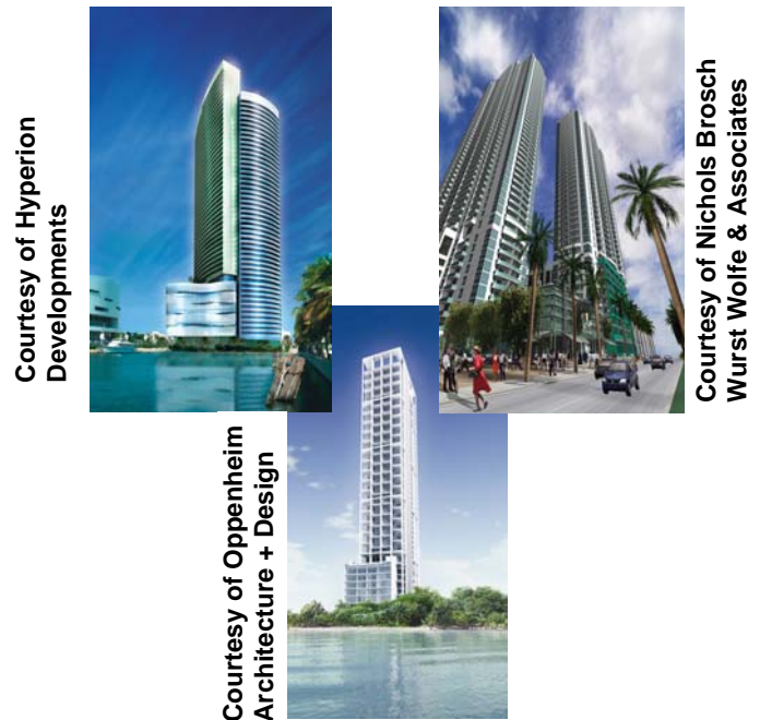
Figure 1 – Typical High-Rise Projects
