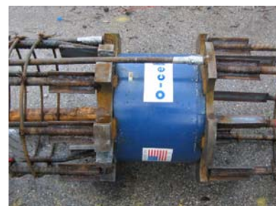
Figure 4 – O-cell installed in rebar cage
