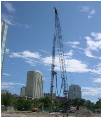
Figure 3 – ACIP Piling Installation
