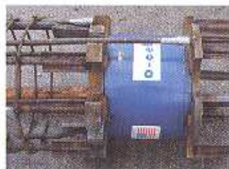
The Osterberg cell assembly (LEFT) was attached to the pile cage and inserted with minimal resistance.
