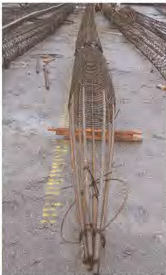
The Osterberg cell assembly (LEFT) was attached to the pile cage and inserted with minimal resistance.
