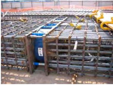
*O-cells are installed within the barrette reinforcement*
