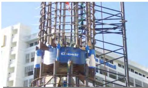
AUGERCAST test pile O-cell assembly ready for placement
