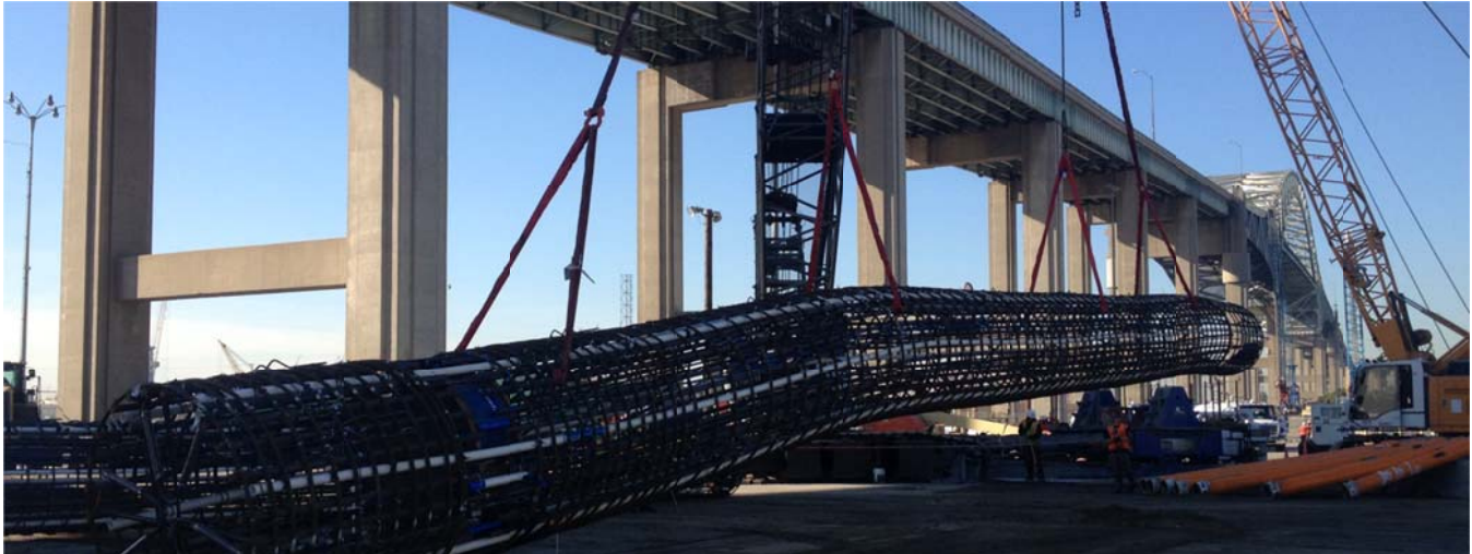
Lifting the Assembly
