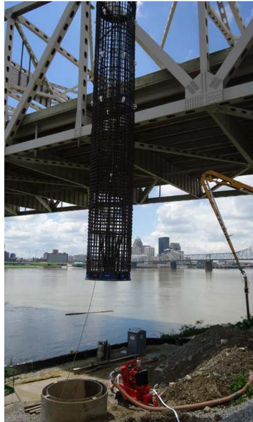
Reinforcement cage installation with O-cells
