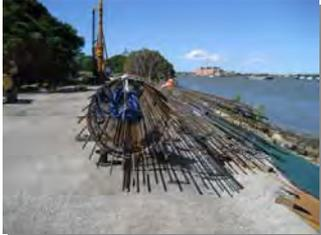
O-cell Assembly ready for lifting
