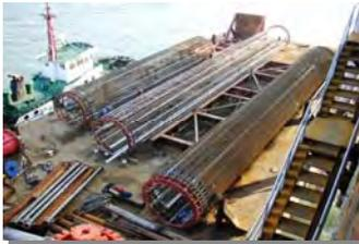
Cage sections in preparation. Several lengths of reinforcing cage had to be spliced together over the bore
