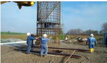
Installation of pile cage with O-cell assembly
