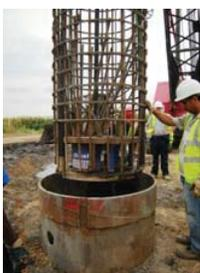
Installation of pile cage with O-cell assembly
