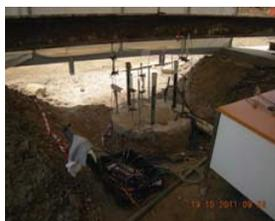
O-Cell Pile test in progress
