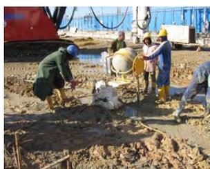
Post test grouting of a working pile
