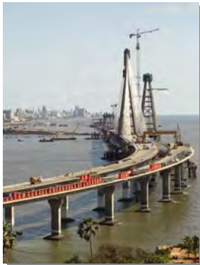
Under construction, May 2008
