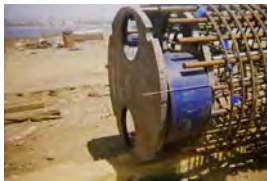
Lower level O-cell arrangement
