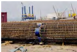
Upper level O-cell arrangement
