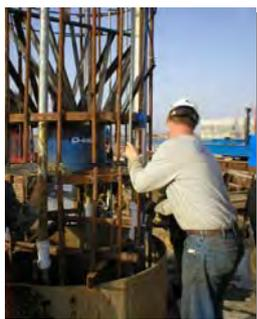
Installation of reinforcing cage with O-cell
