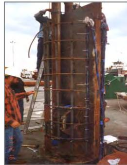
An O-cell assembly is prepared for installation using two 4 MN (900 kip) cells for use in a 1200 mm (48") diameter shaft.
