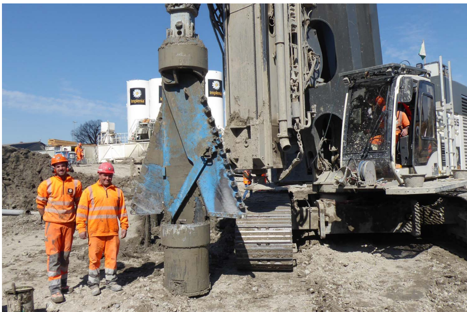
Figure 6. Expanded drilling tool diameter 1850 mm (6 ft) attached to drill rig (Implenia)
