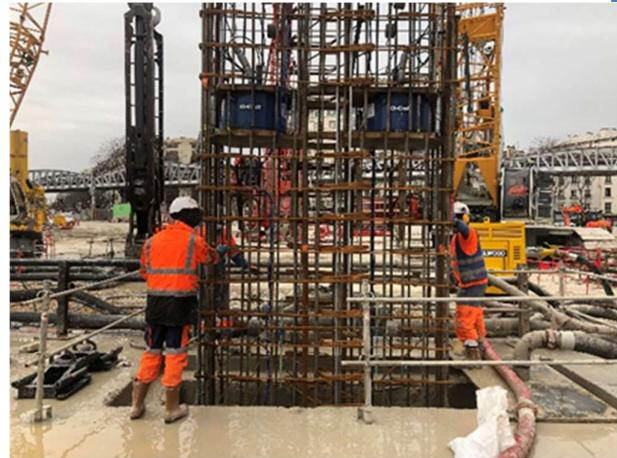
Fig. 4. Insertion of the reinforcement containing the O-cell assembly.
