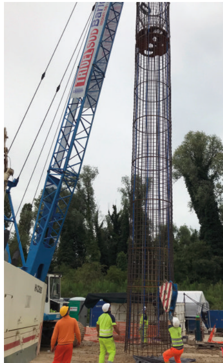
Handling a reinforcement cage with built-in O-cells
