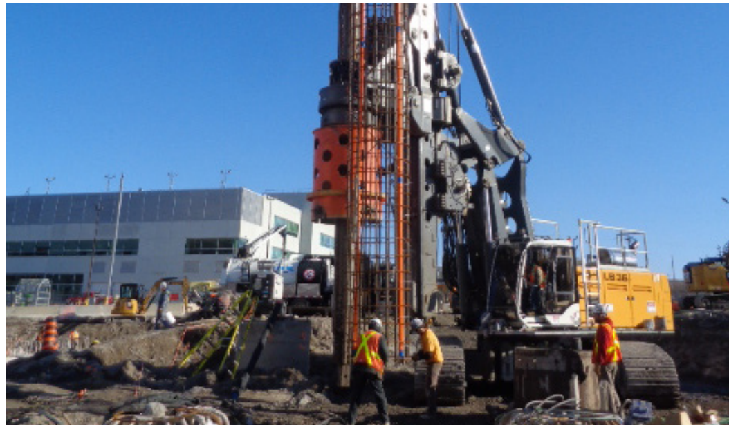
Installing the cage assembly
