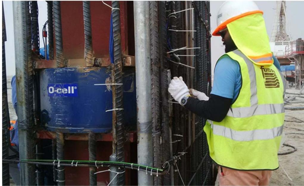
Installation of reinforcement with O-cell arrangement
