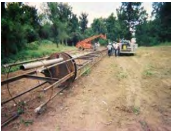
1 of 8 O-cell tests ready for placement
