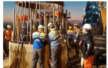
Preparation being carried out to protect Osterberg Cell instrumentation before lowering cage to final elevation
