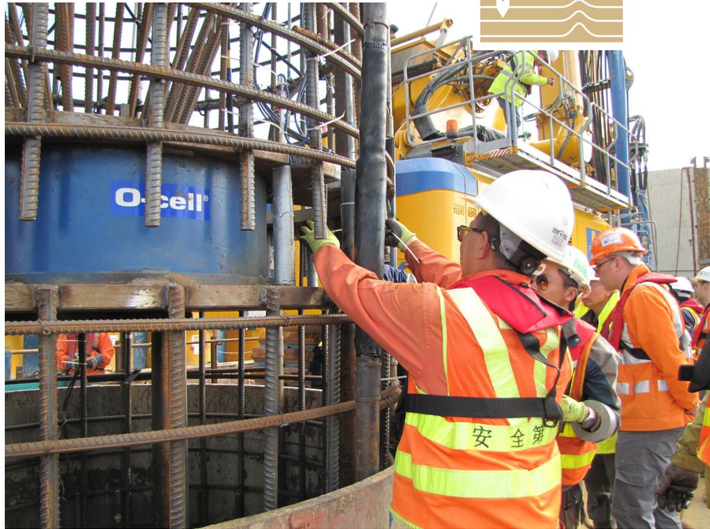
Inspection of loading assembly before cutting Osterberg Cell protection straps required during cage lifting operation
