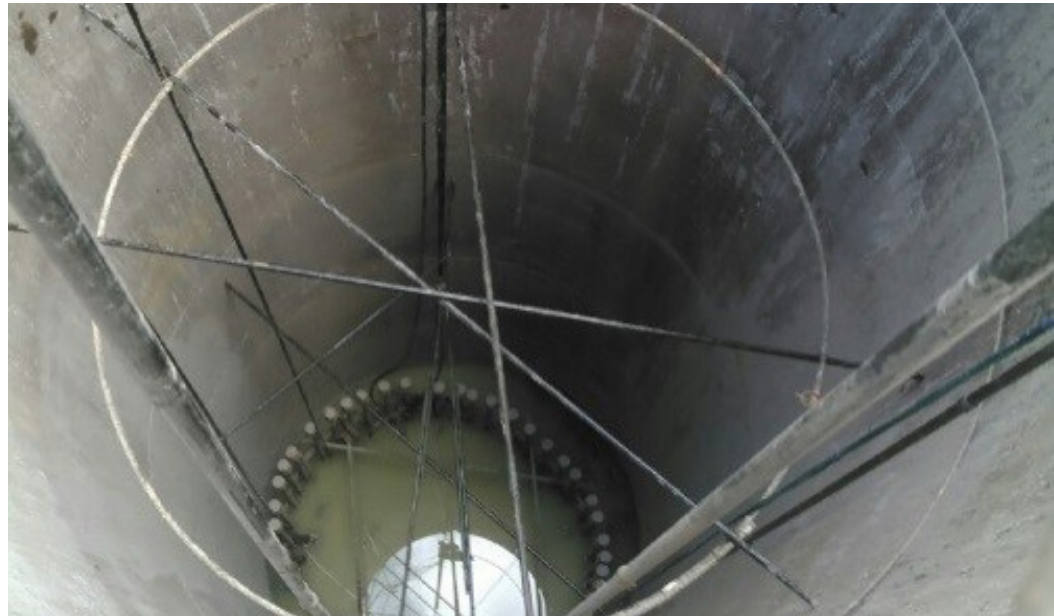
120-inch Diameter Steel Temporary Casing
