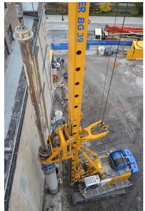
Secant pile wall under construction
