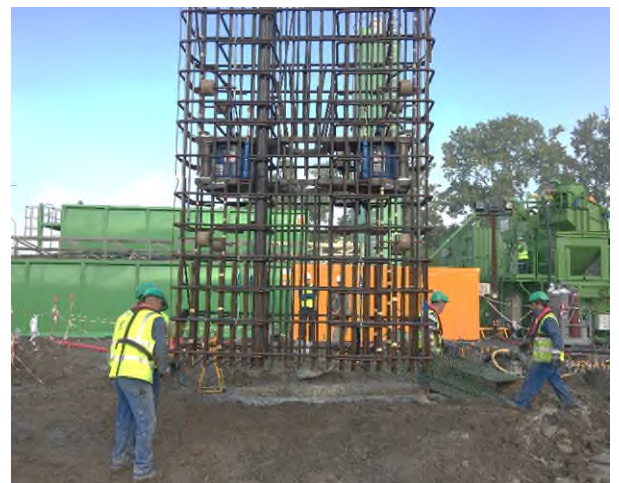
Installation of the reinforcing cage and instrumentation into the panel
