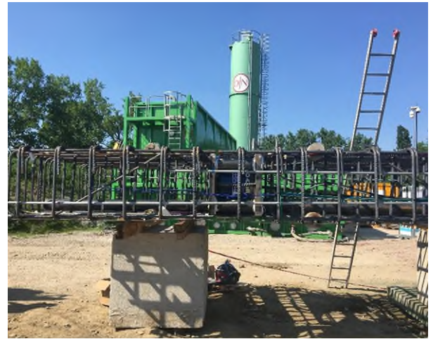
Assembly of the O-Cell® arrangement into the reinforcing steel
