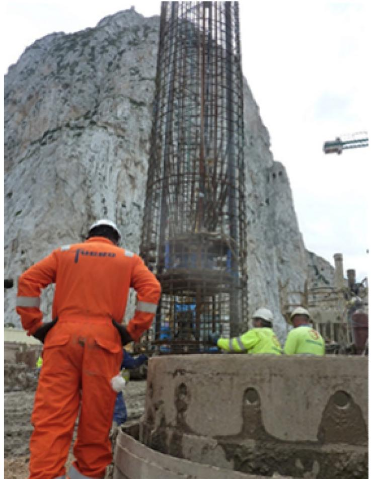
Reinforcing cage, O-cell® and instrumentation ready for installation into the pile bore
