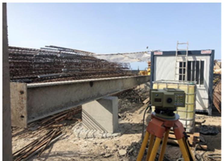
O-Cell® test in progress. The steel beam is for reference only
