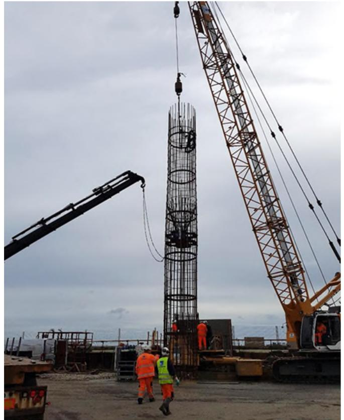
Reinforcement with O-cell during installation
