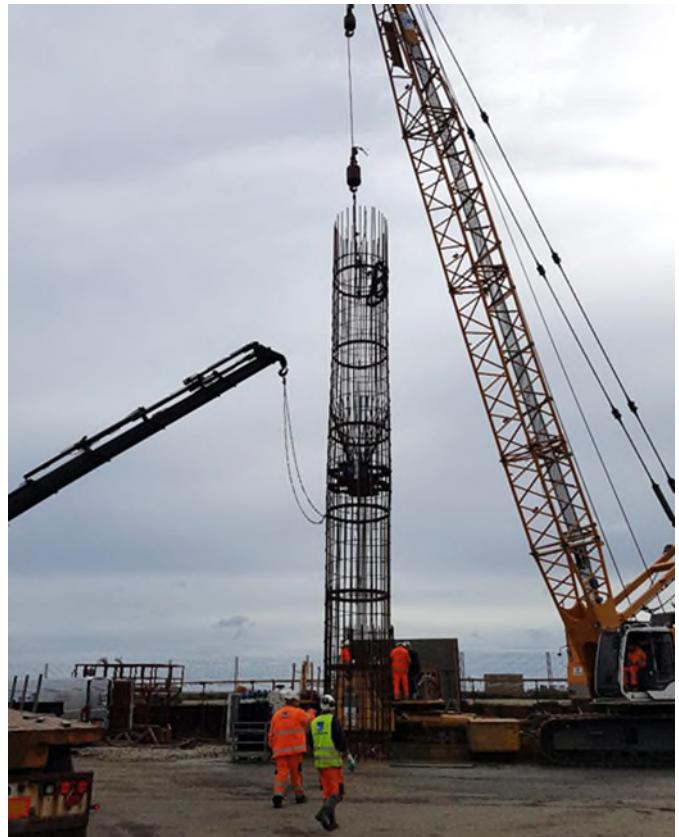
Reinforcement with O-cell during installation
