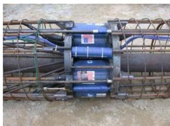
Assembly of 2x330mm O-cells in Ø880mm pile, pre-fitted with a concrete tremie pipe Gönyü, Hungary
