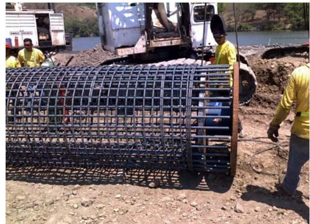
Completed production rebar cage with O-cell
