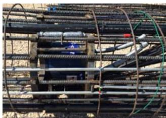
O-cell placed 2 m from the bottom of a Ø1200mm pile, mobilising 18MN
