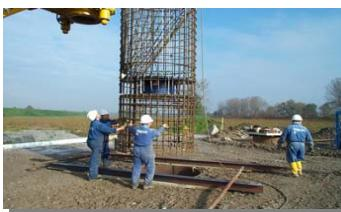
Installation of pile cage with O-cell assembly
