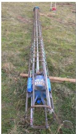
Reinforcing cage, O-cell and instrumentation ready for Installation
