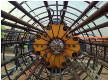
O-cell Assembly in Working Pile
