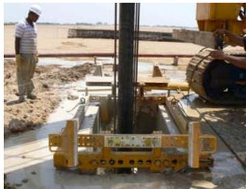
Construction of the barrettes using hydroraise and bentonite slurry
