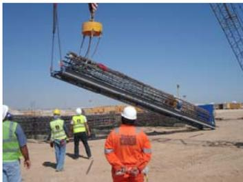
Lifting of O-cell Cage under supervision of Fugro Loadtest Engineer
