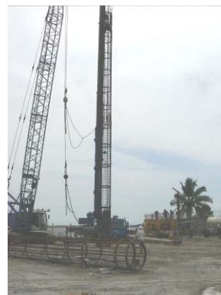
Multi-level O-cell cage ready for installation
