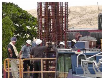
Pile reinforcing cage for TP02, with O-cell and grout pipes, being installed
