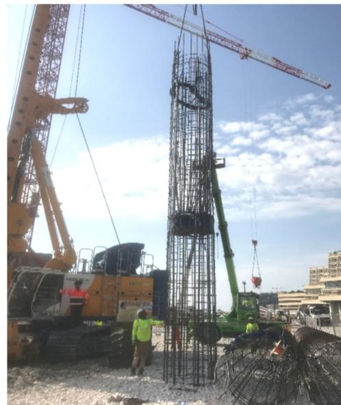
*O-cell cage lifting into place for installation into the pile bore*
