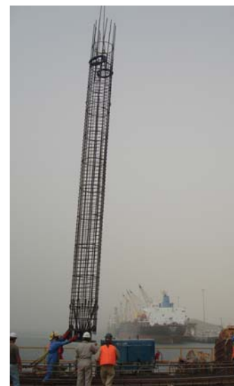
Cage Installation in Progress
