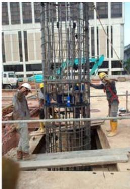
Installation of O-cell assembly through the existing multilevel underground car park.
