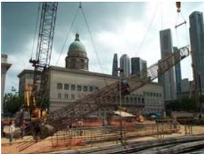
Placing cages within excavation through existing basement car park
