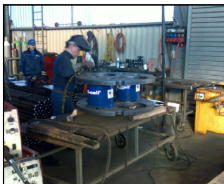
O-cells assembly at the cage fabrication yard
