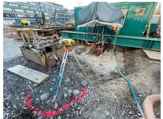
O-Cell® test in progress.
