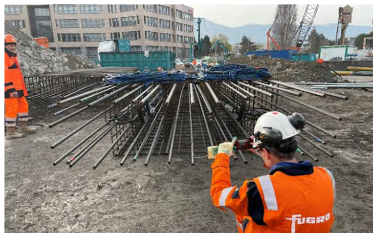
Reinforcing cage delivered to site ready for installation
