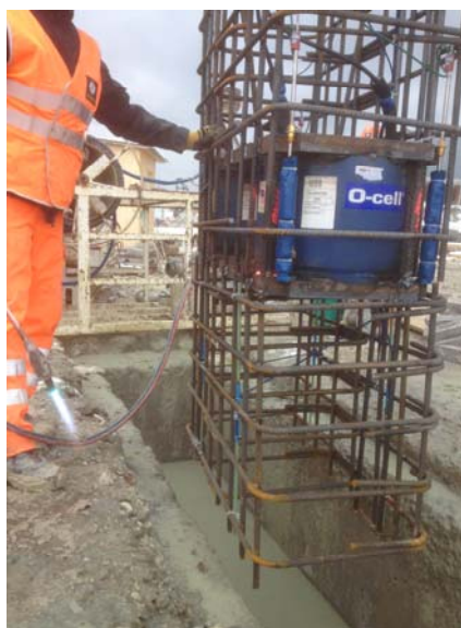
Installation of reinforcement with O-cell arrangement
