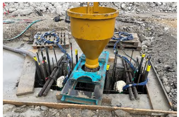
Concrete tremie pipe ready for filling the panel
