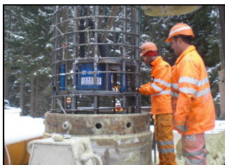
Installation of the cage with two 405mm O-cells
