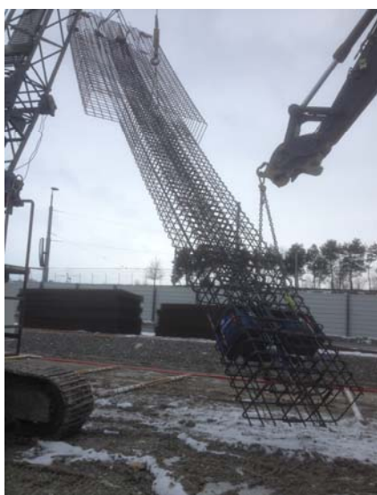
Lifting of the "T" shaped reinforcement
