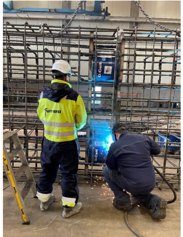
O-Cell® cage assembly in the factory
