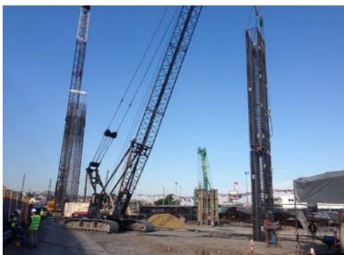
Cage placement with O-Cell assembly
