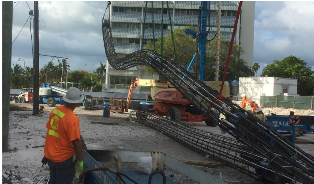
Preparing foundation construction
