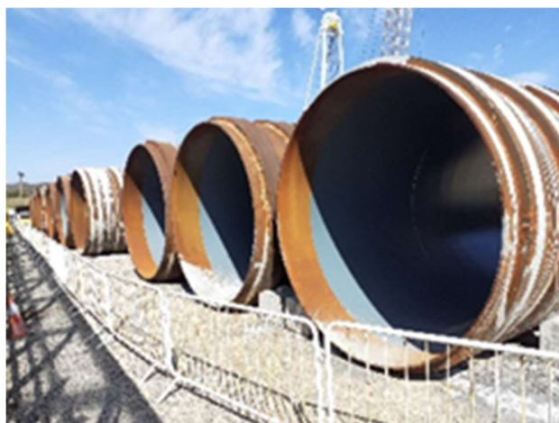
Shaft casings ready for installation
