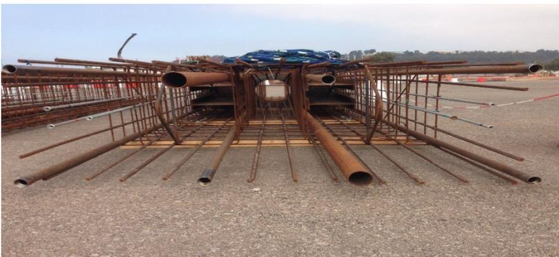
Full scale bi-directional static load testing using Osterberg-cells was utilised as the method which is specifically appropriate for the high test loads required on barrettes of this size and bearing capacity. The results obtained allowed confirmation, and potential optimisation, of the foundation design without the need for costly and time-consuming installation of reaction shafts used in traditional top down load testing.
