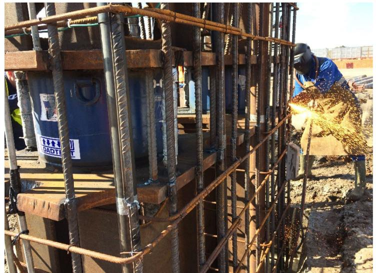
*O-cells positioned within their bearing plate assembly.
