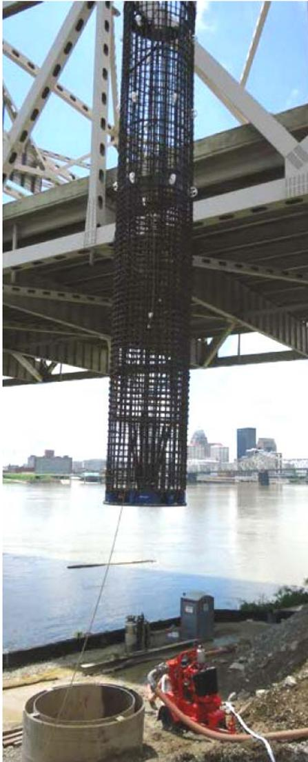
Reinforcement cage installation with O-cells
