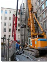
Installation of the bottom section of reinforcing cagewith both O-cell arrangements
